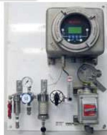
The IR-1150 is a high-pressure sampling system designed to remove particulates and condensed vapors from the emission that petroleum companies, refineries, and transfer station are federally and locally required to monitor. This state-of-the-art sample conditioner features a two-filter sample system that is complete with a pressure regulator, flow meter, and calibration gas selector valve.
